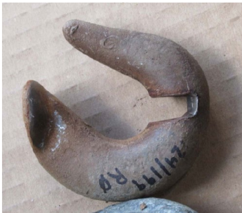
A worn C-hook, like the one pictured here, broke on Nov. 8, 2018, dropping a high-voltage line and sparking California's deadliest wildfire. | PG&E
