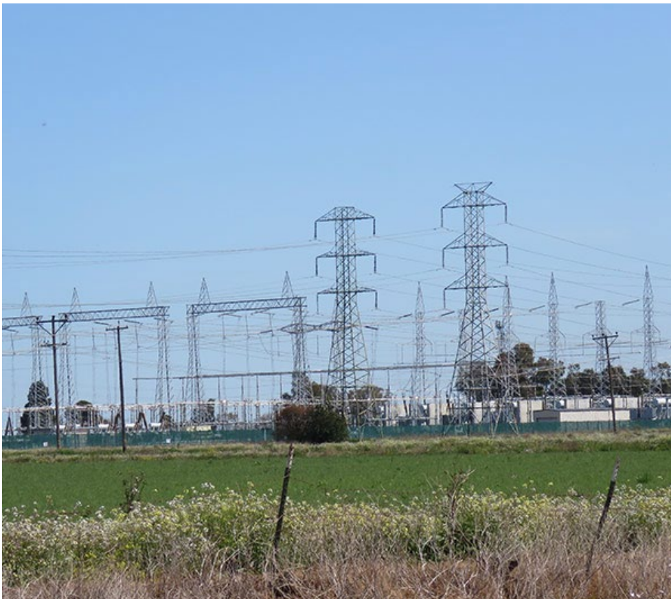
PG&E substation near Dixon, Calif. | © RTO Insider
