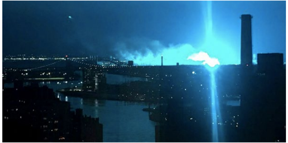
A December 2018 transformer explosion at a Consolidated Edison substation in Queens, N.Y., caused a power outage at LaGuardia Airport. | Con Ed
